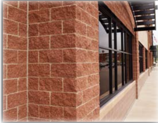
Concrete Masonry Unit with Rockface Finish
