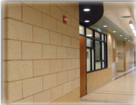
Concrete Masonry Unit with Burnished Finish
